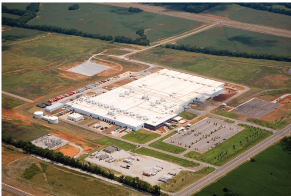
Toyota car plant, Burnaston, 2006 (under development)
